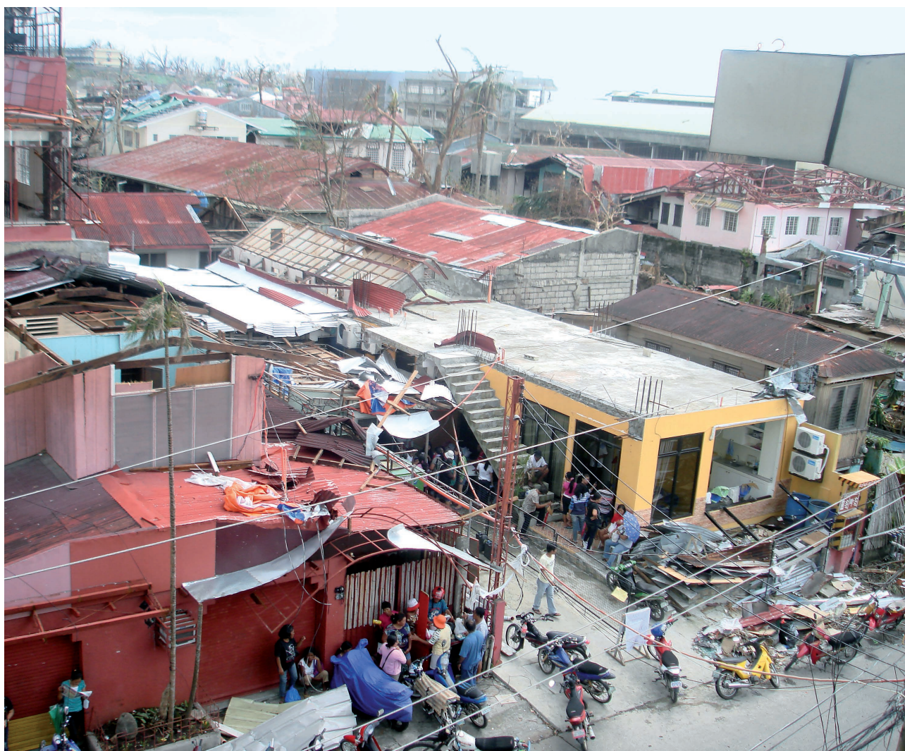
Ormoc City the day after super typhoon Haiyan; OCCCI's laboratory and medical clinic (yellow one-storey building) is completely damaged.
